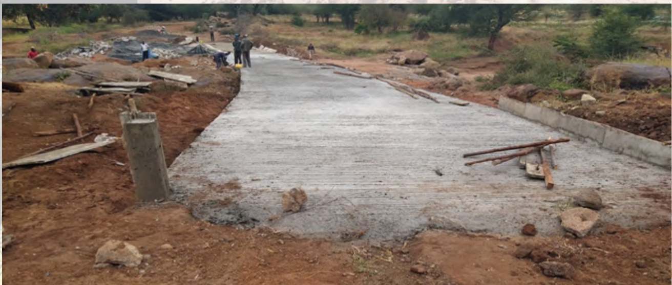
Kanyililya drift slab at Nguu/Masumba Kibwezi West
