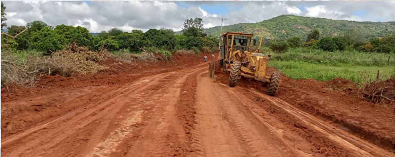
Mechanical opening and grading works along Mituvu-Kandulyu-Ngovu road in Kako-Waia ward -7.2kms
